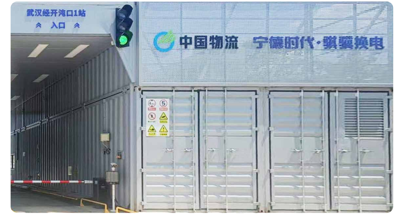
Construction of Battery Swap Station at the Manufacturing Plant
